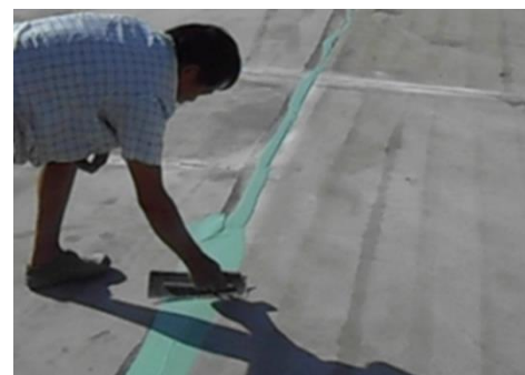
Seal the crack by trowel
